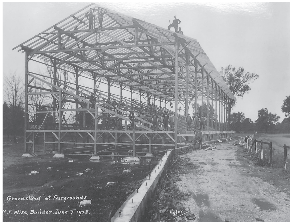
1928 Building the New Grandstand
